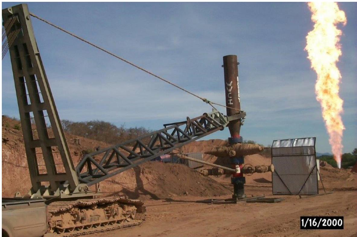
Figure 1: A single blind ram capping stack is prepared for installation over a high rate gas well. The capping stack lies above a diverter spool with outlet valves installed. Reproduced courtesy of Wild Well Control.
