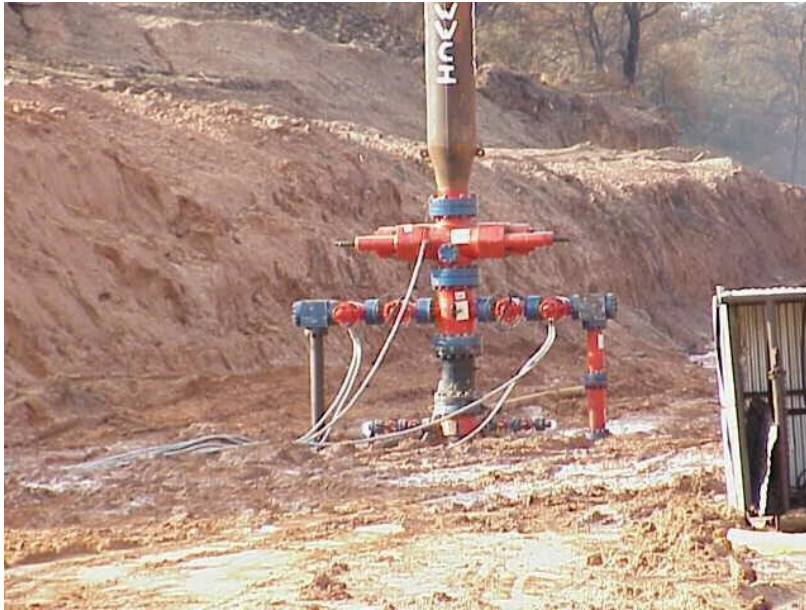
Figure 2: The capping stack installed over the incident well with hydraulic lines installed and well shut in. Reproduced courtesy of Wild Well Control.
